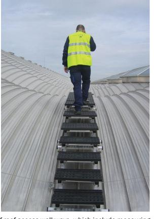
EN516:2006 is the European standard for the test requirements of roof access walkways, which include measuring the deflection and residual deformation under specified loads. These criteria have been surpassed in all testing and as this is a harmonised standard allows the system to be CE marked under the European Construction Products Regulation No. 305/2011.
